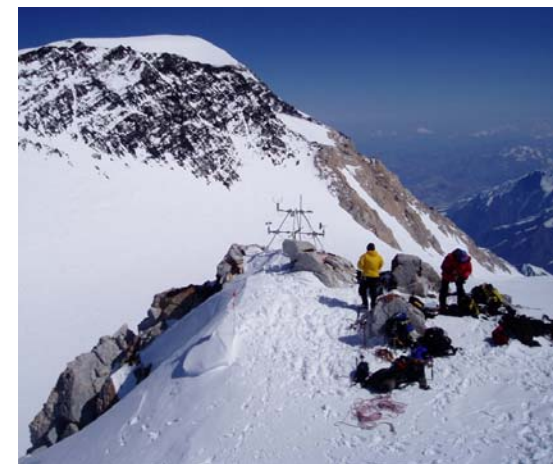
Servicing the UAF/IARC weather station on Mt. McKinley (just below the summit at 18,700 feet). Photo by Tohru Saito (IARC), members of the Japan Alpine Club assisting.
